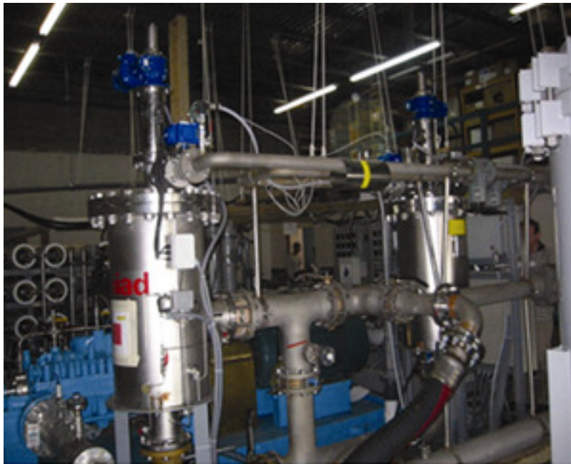
Using an automatic self-cleaning screen filter to remove suspended solids before water reaches its RO membranes, this Virginia desalination plant uses its fine filtration more efficiently.
