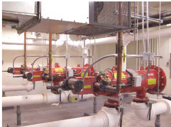
Figure 3: Removing suspended solids at the point of entry of domestic water reduces plugged aerators, showers, and toilets in high-rises, and protects delicate medical machinery and patients in healthcare facilities.
