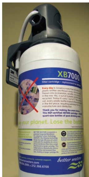
An XB7000 POU filter combines a membrane and activate charcoal for 0.2-micron filtration. It is safeguarded by a screen filtration system at the water supply's point of entry.
