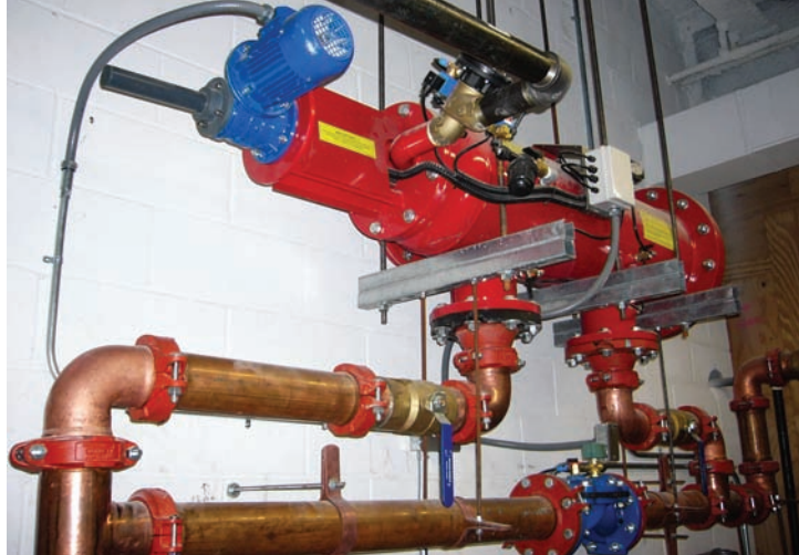
Requiring minimal power and less than one percent of the total flow for back flush, this automatic self-cleaning screen filter captures sediment and scale at the water supply's point of entry, before it becomes a quality or maintenance problem upstairs.
