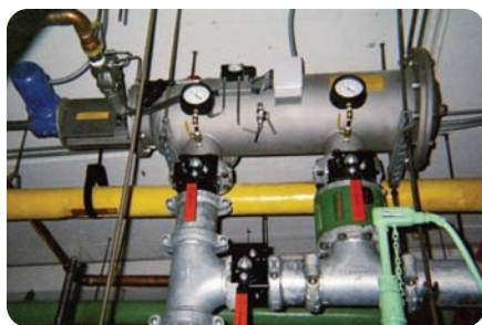
Point-of-entry filtration allows developers to build “greener” and protect apartments (or hospital rooms) from clogged aerators and showerheads.
