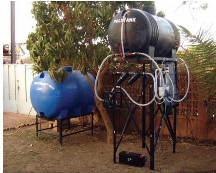
McGuire's water purification system includes two degrees of filtration and a sidestream chlorination system that uses electricity and table salt to disinfect entire tankfuls of water.
